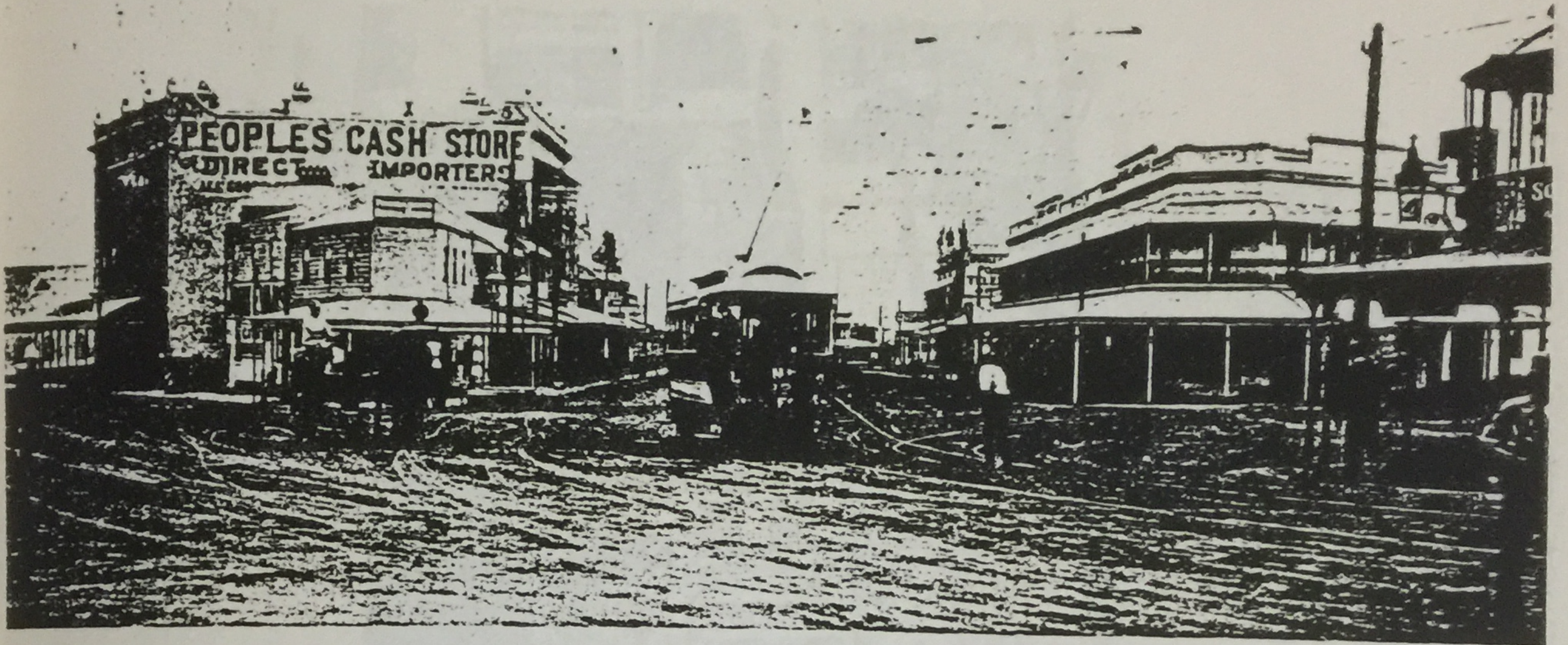
The first Woolloongabba Post and Telegraph Office in Logan Road (figurines on top) opened 23.9.1889, with electric tram No. 92 Logan Rd - New Farm outbound.
